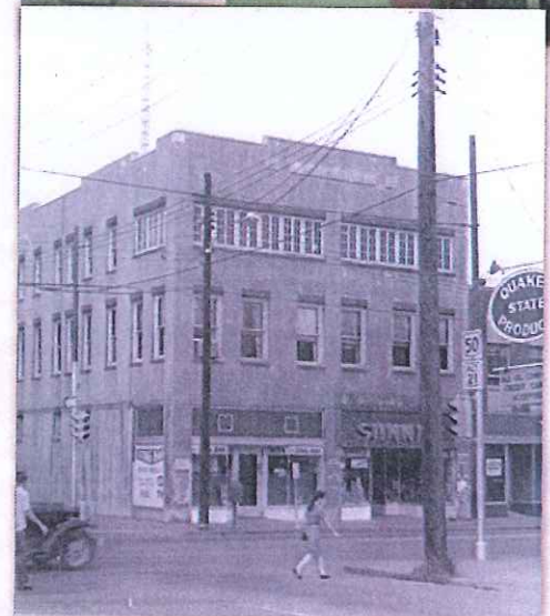
The CVB office building was constructed in 1922 with three stories. The second and third floors were later removed.
